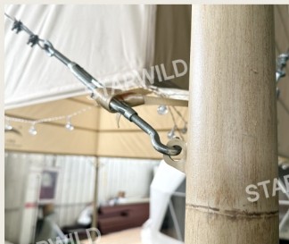
Brace Fixing Point
